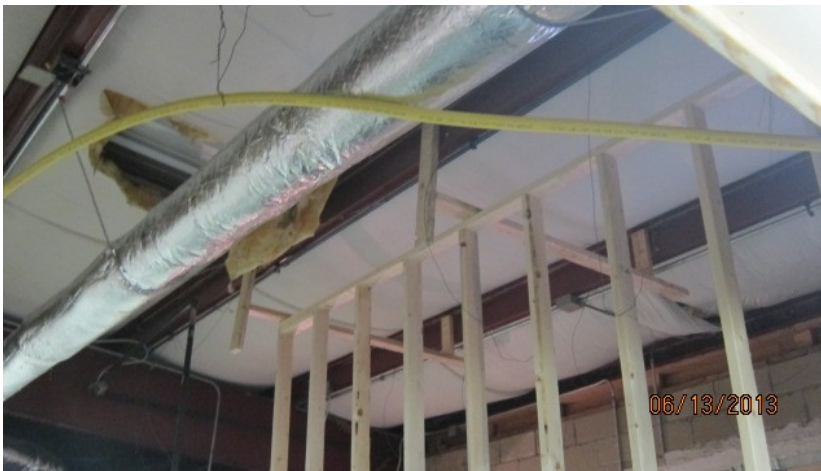
Joe Giampoletti has taken the lead in the Hall kitchen's most recent improvement. The once-leaky kitchen is now leak free.
