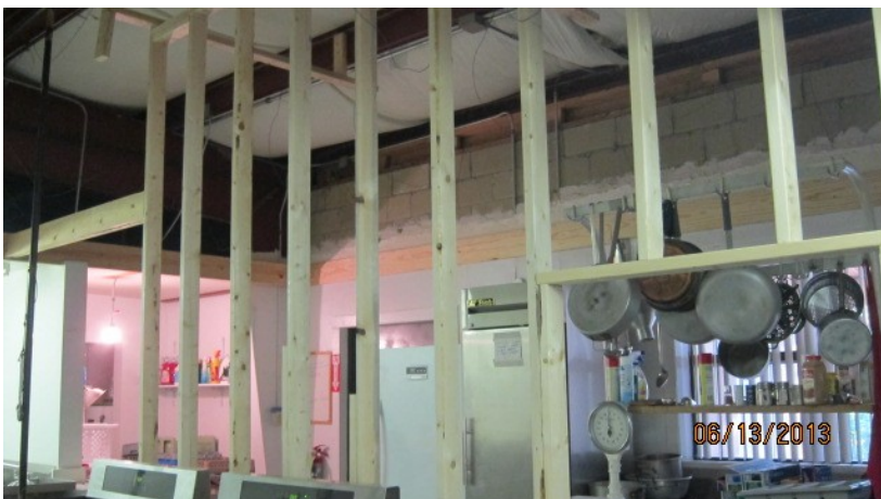
As Joe and his helpers await the new vent-a-hood for the dual ranges, new shelving is being constructed. Those hanging pots and pans will soon have their place on shelves.
